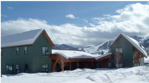
(top) Deep overhangs and deciduous trees provide shade from intense Colorado sun. Low-maintenance exterior materials like cement siding and composite decking are specified. (Photo Source: Ed Hancock, National Renewable Energy Laboratory)
